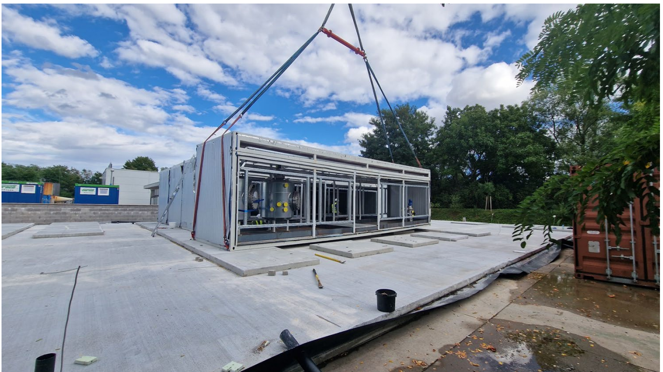
Positioning of the prefabricated containers at the Sorption-Demo Plant in Landau, Germany.
